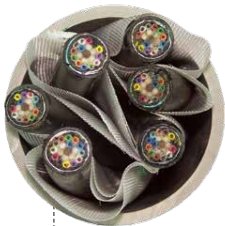
4" 3-Cell packs with 6 1" OD cables in 4" conduit
