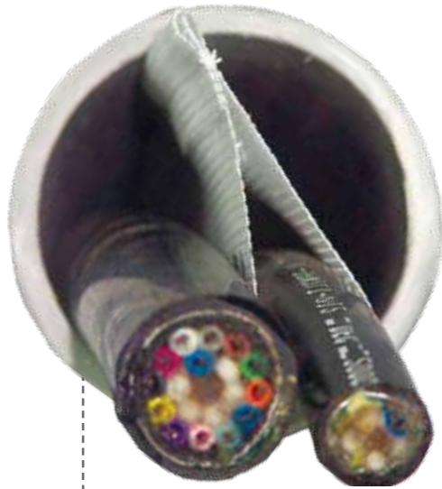
2" 1-Cell MaxCell overriding incumbent cable in 2" conduit
