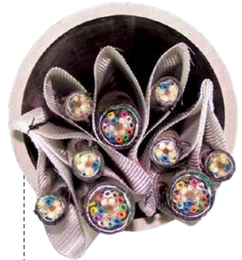
3" 3-Cell packs, 9 cables in 4" conduit
